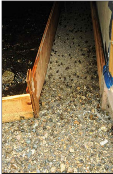
Toadlets were redirected under Highway 31A with infrastructure built to avoid a close-call high mortality situation amidst Slokan Valley wildfire evacuations.
